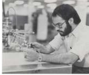
Figure 33. Pulling Lamps Off Vacuum System
